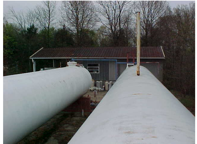
Retrofit to 50 year old LPG tanks
