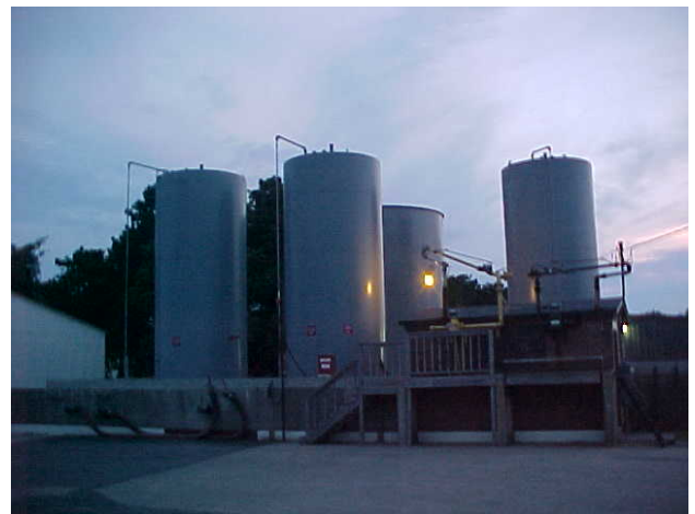
#2 Fuel Oil Tanks with obscured view to largest tank
